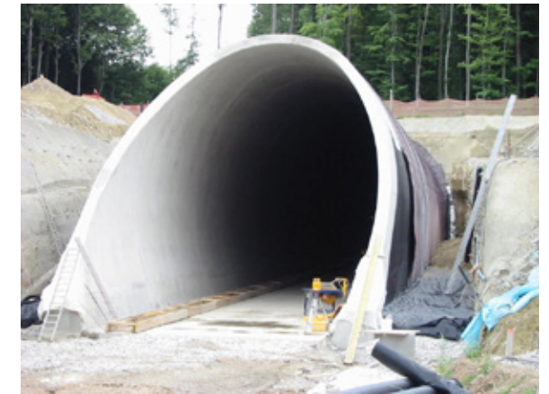
Cut and Cover Tunnel Application.
